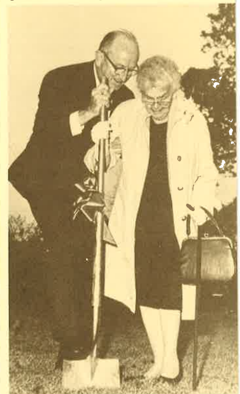
George W., Peacock Jr. and resident Lois Keith (100 years old) at Florida Christian Apartments ground breaking
