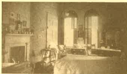
A room in the "Old People's Home," (1902)
